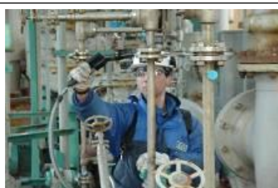
Figure 3.37: Leak concentration measurement
