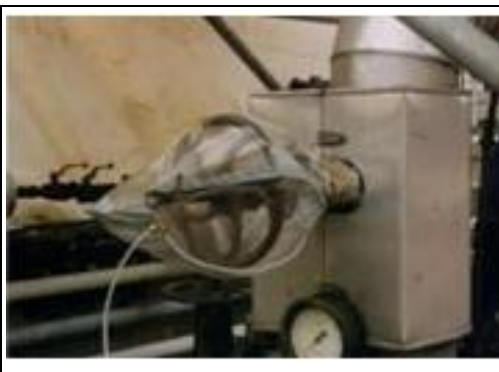
Figure 3.38: Bagging of a leaking valve
